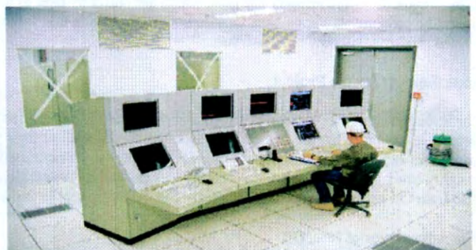
Inside the control room
